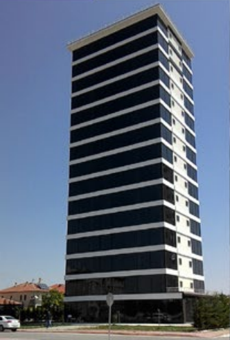
2000 m 2 Hava Kaynaklı 120 kW Cam Kule Airport Residences 52 Oda / Kayseri
